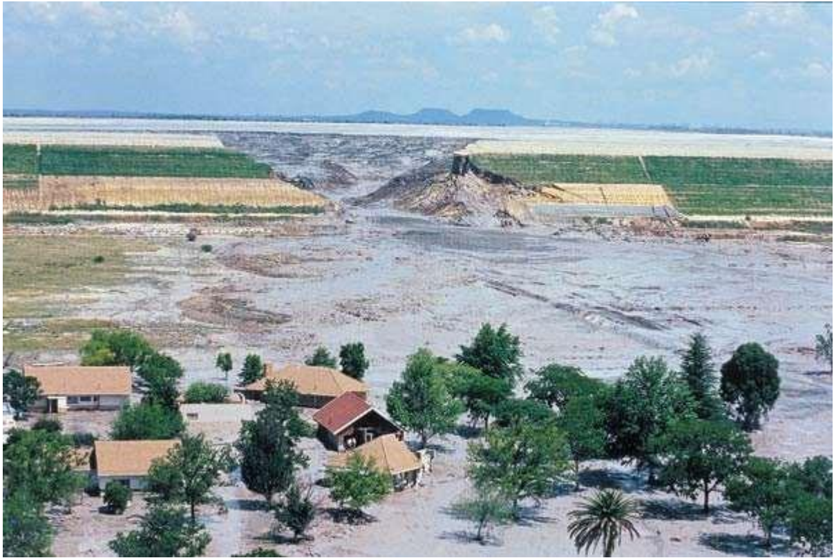
Figure 13: Image of the Merriespruit tailings dam failure. (Image from Tailings.org)
