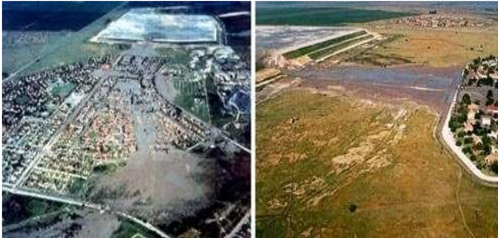
Figure 15: Tailings sweeping through the town of Merriespruit. (Source at tailings.info)
