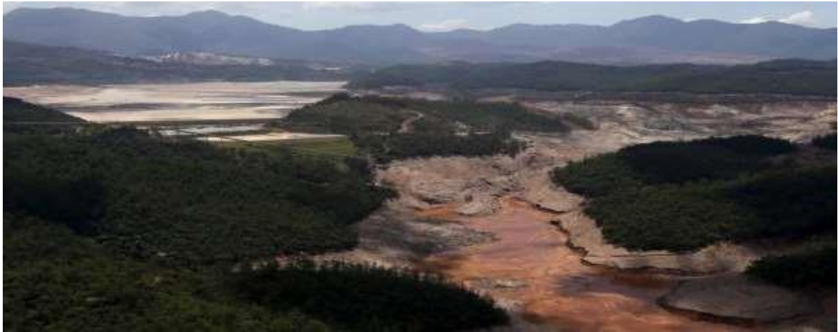
Figure 6: The left hand dam above is intact, whilst the one to the west appears to have failed. (Image by Reuters)
