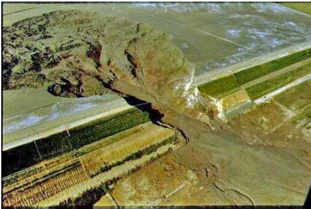
Figure 14 Aerial view of the dam breach. (Source at tailings.info)
