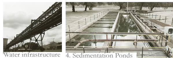
Water infrastructure 4. Sedimentation Ponds
