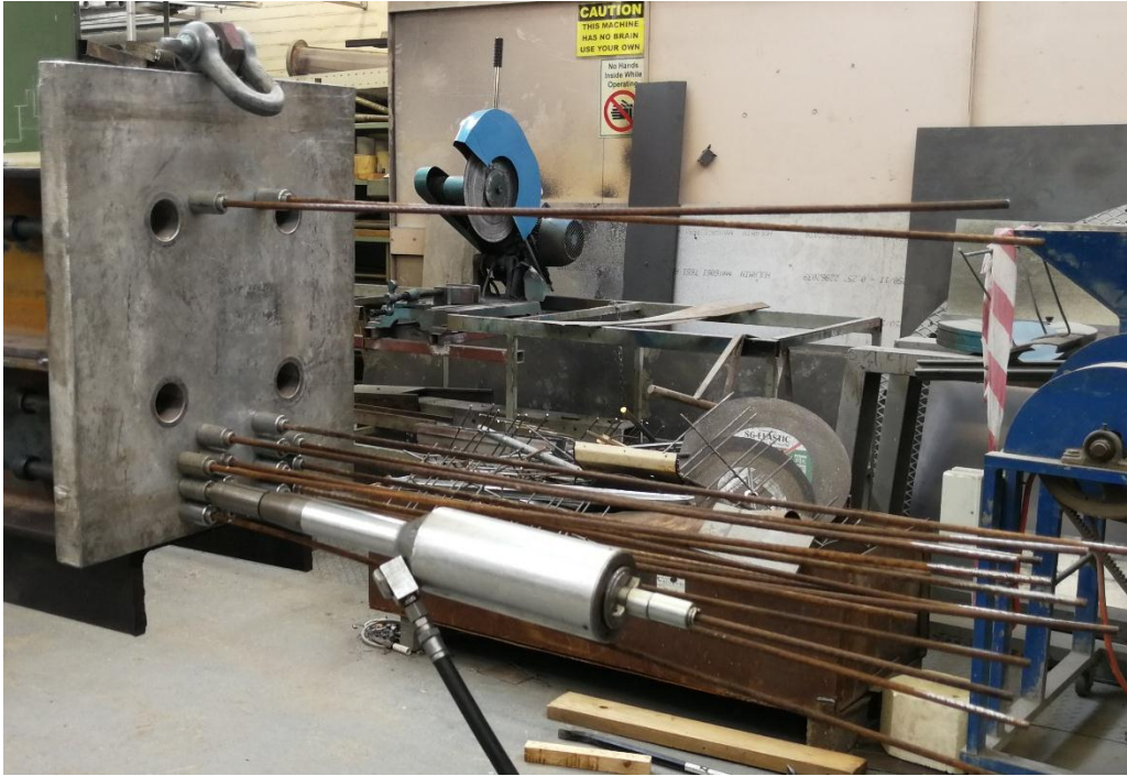
Figure 7.3 Procedure of prestressing the steel wires in large-scale UHPFRC prestressed beams
