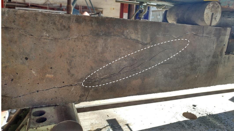
Figure 6.8 Loading cracks as an extension of pre-existing cracks in UHPC prestressed 1m-beams
