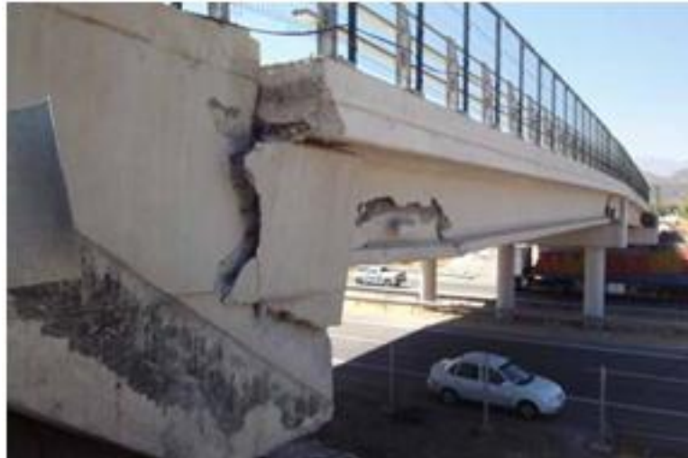
Figure A.1 Curtain wall shear failure at abutment of Chada Bridge (Chen et al., 2010)
