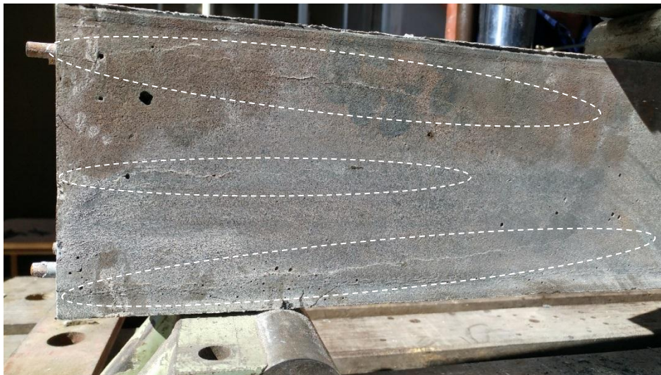
Figure 6.7 Pre-existing cracks due to wire releasing process
