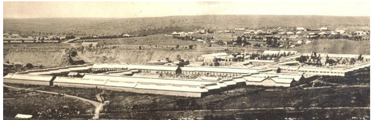
Figure 2.4 - Workers compounds - (Lincoln: 2011)
