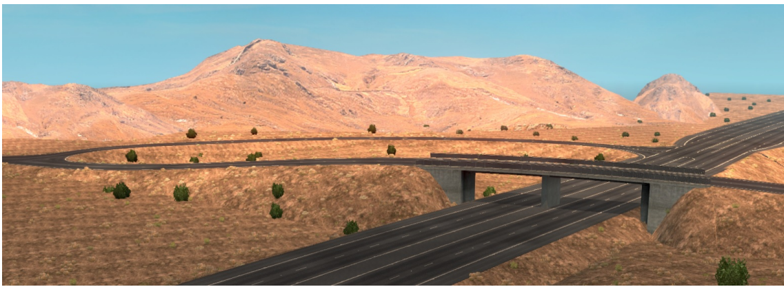
Figure 4.7: Additional view of the N1 and N10 intersection mapped in SATS .
