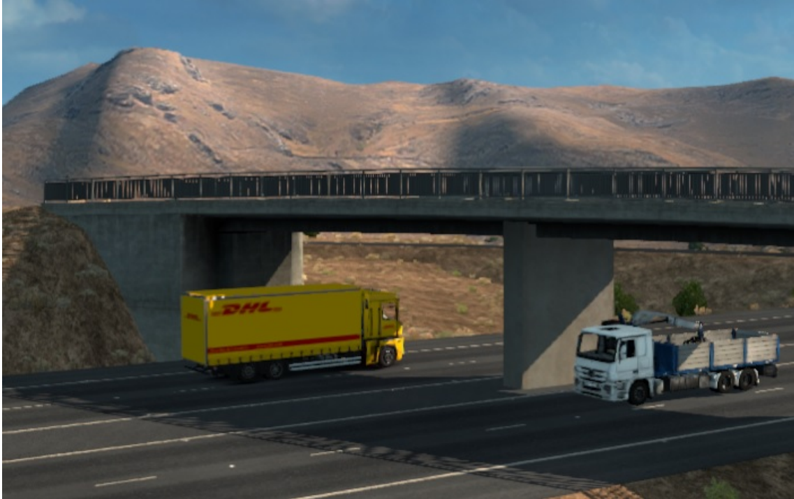
Figure 3.2: Bridge of height 8 m as mapped in SATS.
