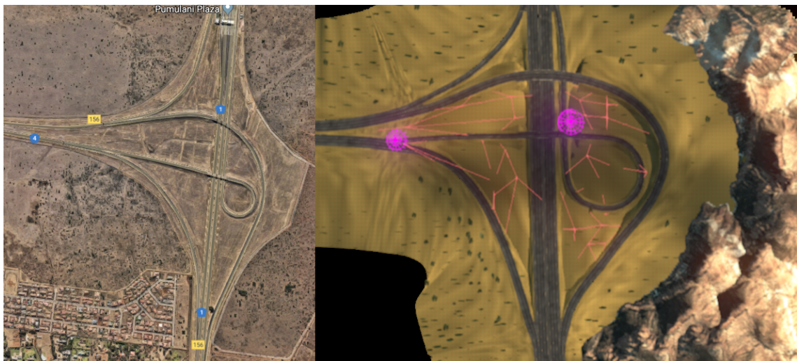
Figure A.6: Top view comparison of N1 and N4 intersection. Source: Google Maps, 25^{\circ}38'45.9'' S 28^{\circ}16'23.7'' E , accessed 25 Augustus 2018.
