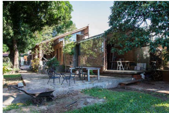
Figure 6-61: House extension with recovered bricks protected by glass sheet (old enclosed in new) (Cairoli 2012)
