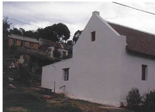
Figure 4-18: Addition to house (De Preez 2009:33)
