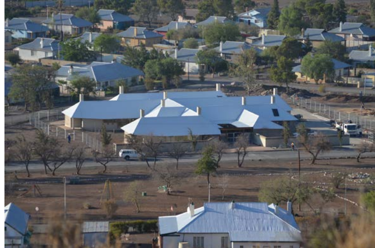
Figure 6-74: Photo of Beaufort West Hillside Clinic with surrounding context (Kuschke & Jehand 2017:33)
