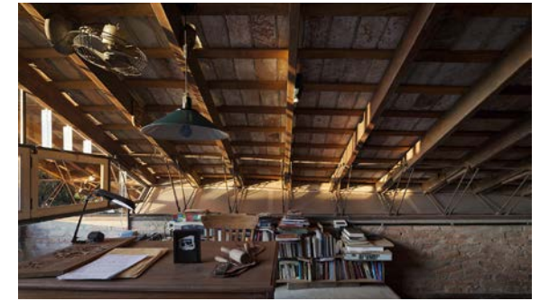
Figure 6-60: Mezzanine floor (Cairoli 2012)
