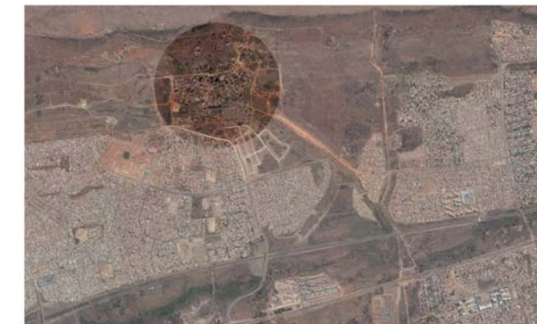
Figure 1-2: Westfort development over time (Author 2018). refer to Appendix C on page 190 for more detailed development over time.
