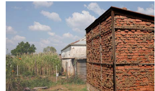
Figure 2-8: Constructing new buildings to accommodate adaptation of Westfort (Swart 2015)
