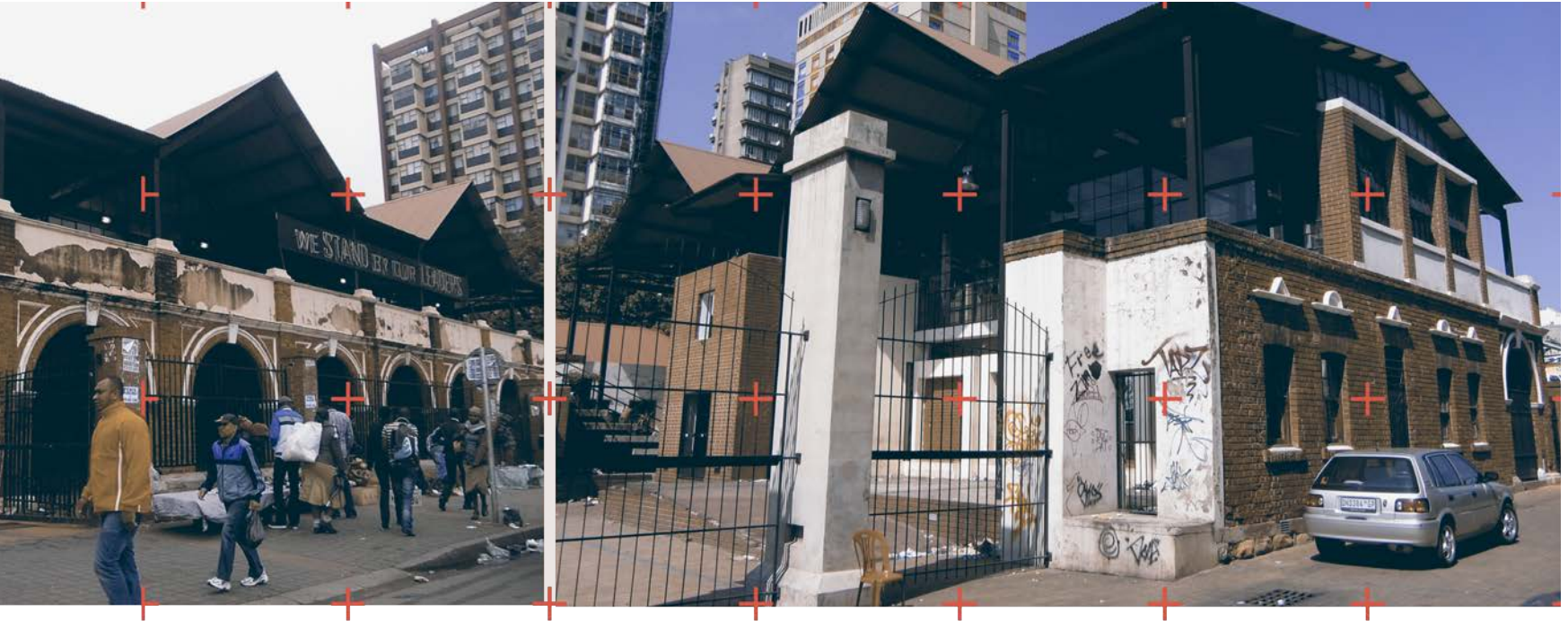
^ Fig. 4.28 - Current external condition of the west building
