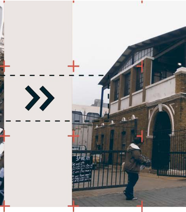
Fig. 4.27 - Current external condition of the west building
