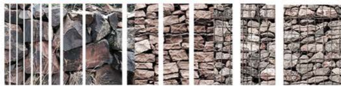
New gabion walls
