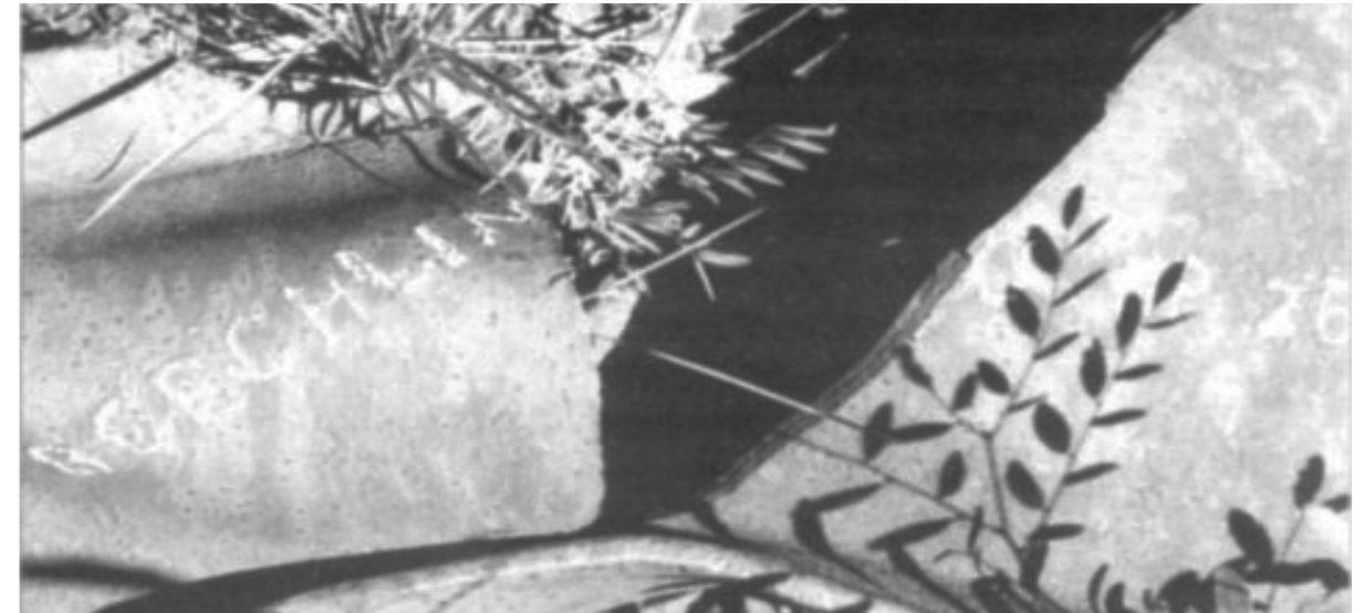
Annotated in the photo above: The beam marked "ROECHLING NR 28"
