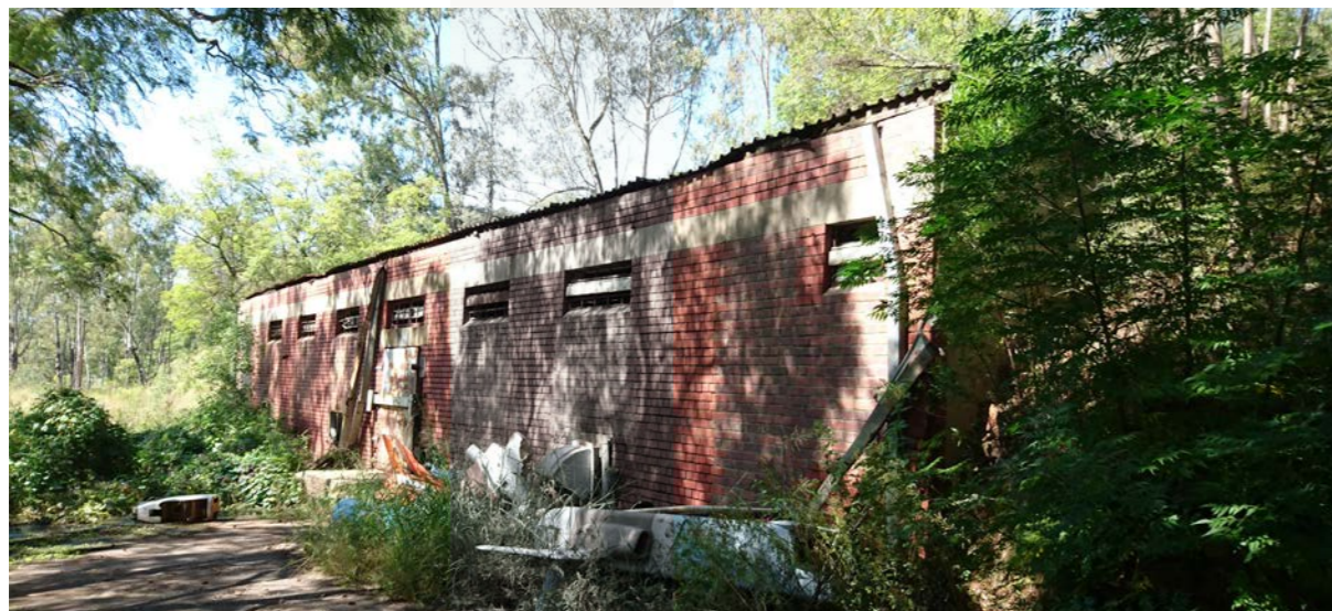
Figure 2.62 The re-roofed flame-tracer building west of the Red Magazine (Author, 2018)
