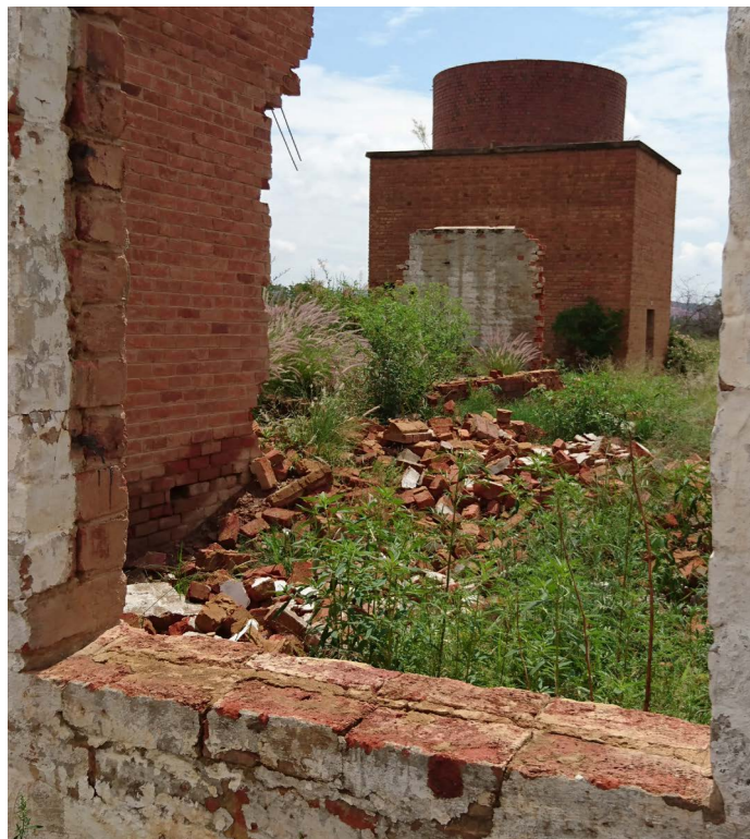
Fig. 01. Above; Photo, ruins of the old Era Brick Factory (Author, 2018)
