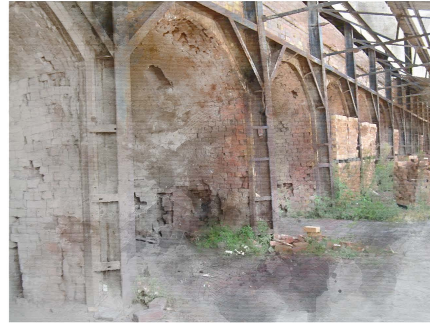
DECOMMISSIONED BRICK OVEN
