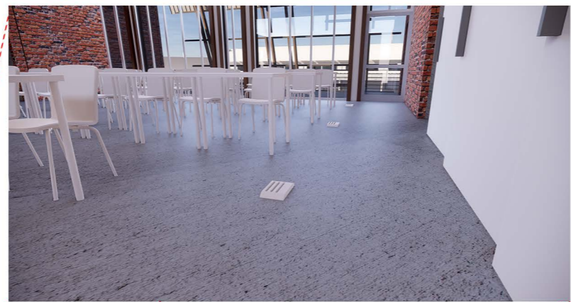
FLOOR VENT TO LET IN FRESH AIR
