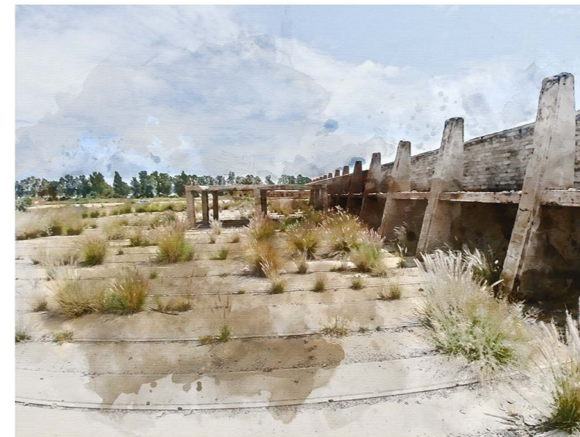
LEFTOVER BRICK DRYING TRACKS
