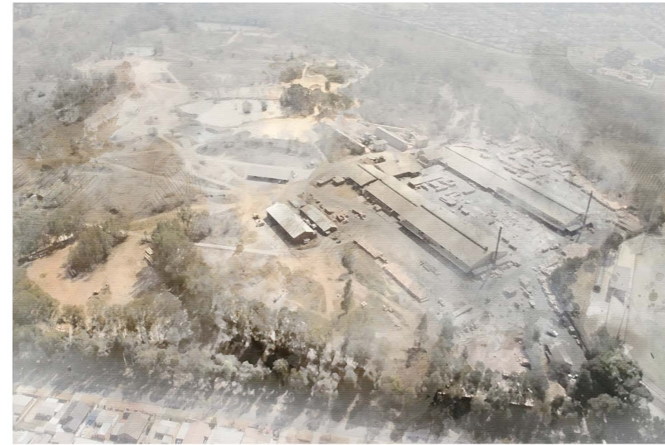
AERIAL PHOTO JUST BEFORE THE FACTORY'S CLOSURE
