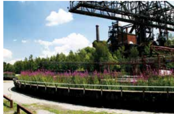
Figure 2.67: Image of the site
