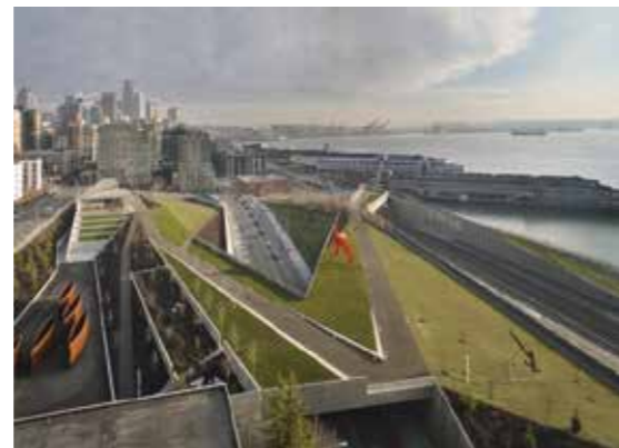
Figure 2.40: Image of the site
