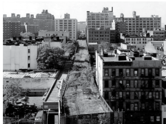
Figure 2.26: Image of the site prior to the intervention
