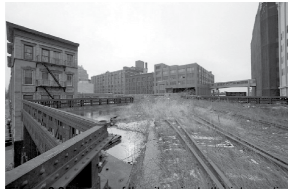
Figure 2.25: Image of the site prior to the intervention
