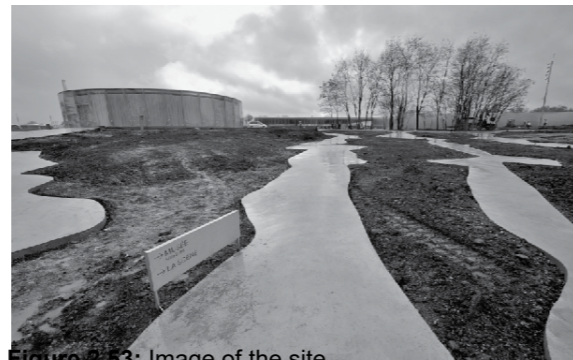
Figure 2.53: Image of the site
