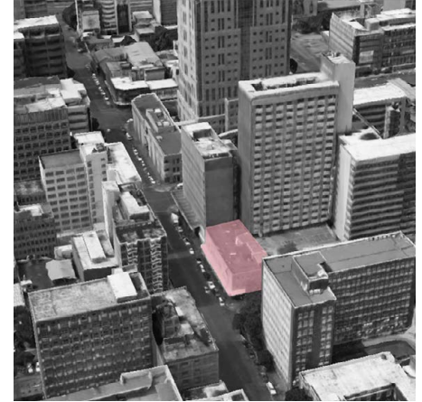
FIG. 2.5.1: Johannesburg Institute of Engineering and Technology, De Beer Street (Google Earth edited by Author, 2018)
