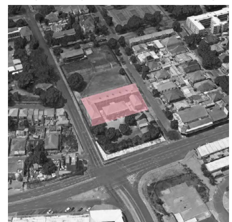
FIG. 2.5.7: Central Johannesburg TVET college, Pretoria St, Troyeville (Google Earth edited by Author, 2018)
