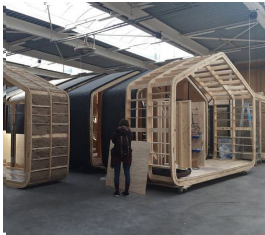
Figure 8.1.3.2 Timber frame before wrapping (Fiction Factory, 2014)
