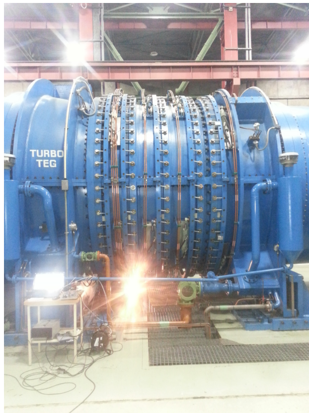
Fig. 16. Side view of the axial compressor on which BTT tests were done. In the bottom left corner the data acquisition and sensor conditioning equipment can be seen.
