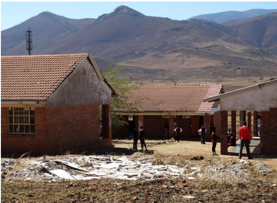
Photograph E2: Run-down school buildings
