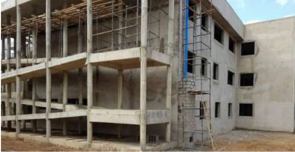
Figure 5.8: Construction of ICT, Library at BTC
