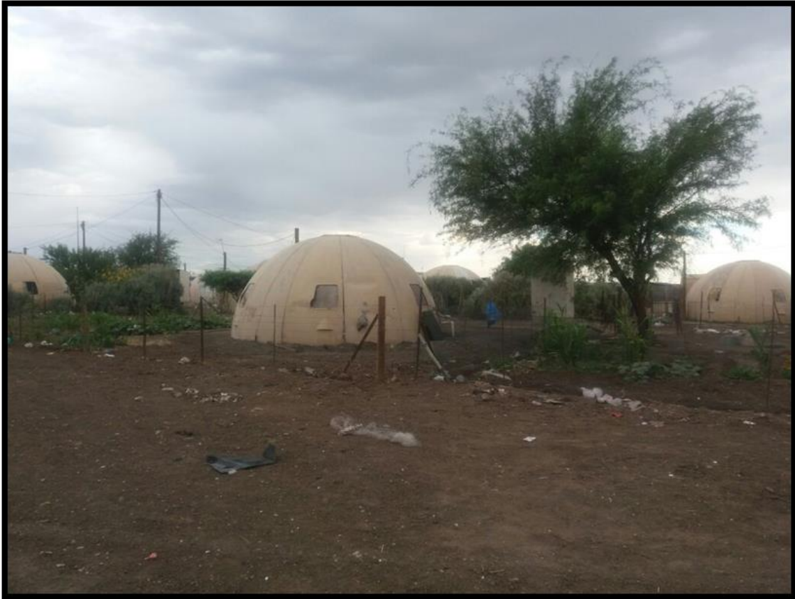
Figure 4.20: Photograph of the 'Pampoene' houses in NCP
