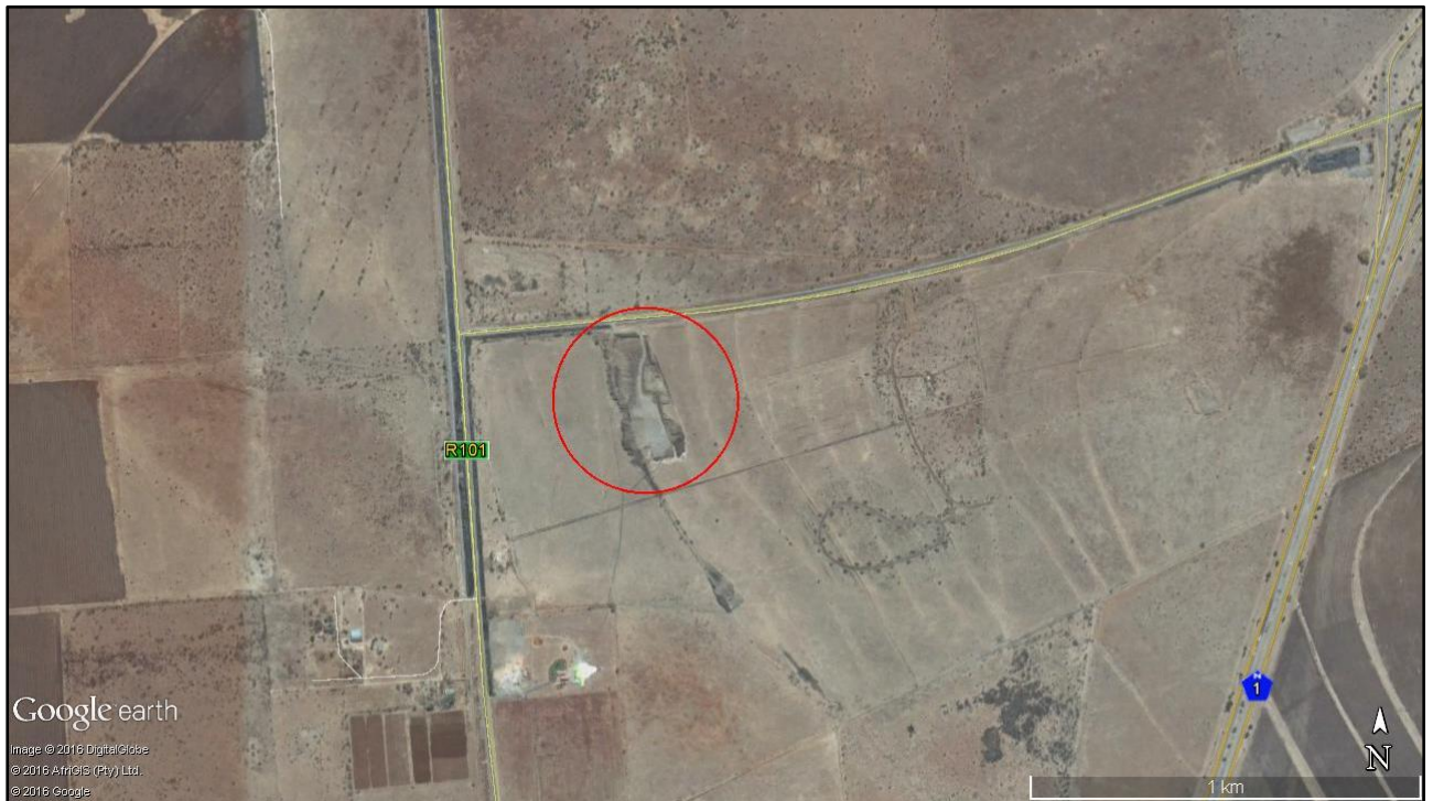
Figure 15: Codrington site on Springbok Flats Basalts, approximate area of investigated quarry (©Google Earth, 2015).
