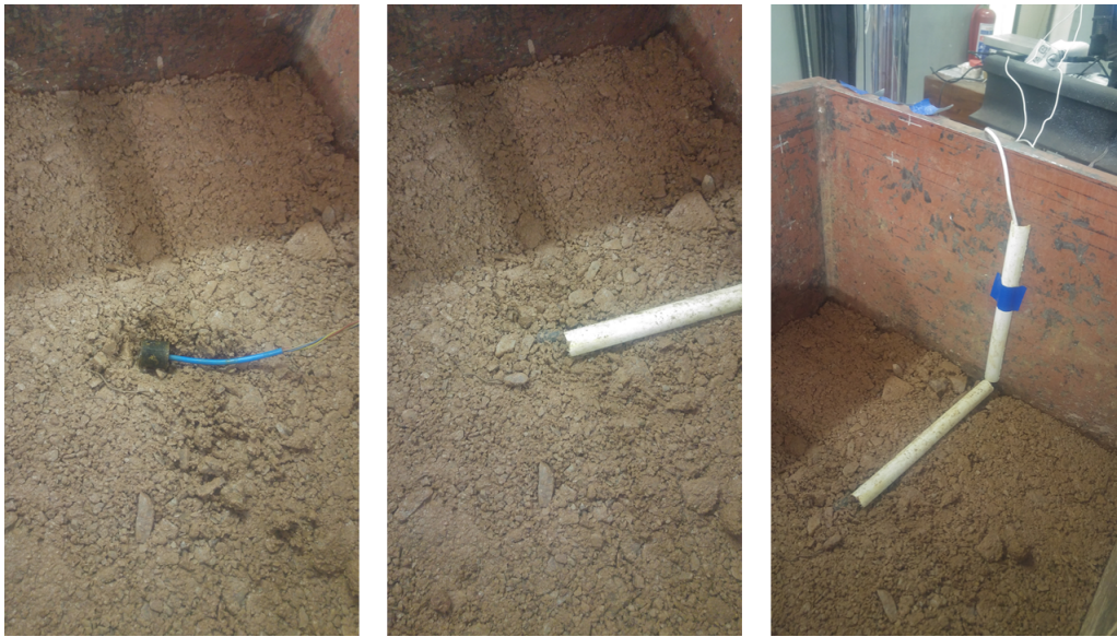
Figure 3.10: Tensiometer installation with cable protection
