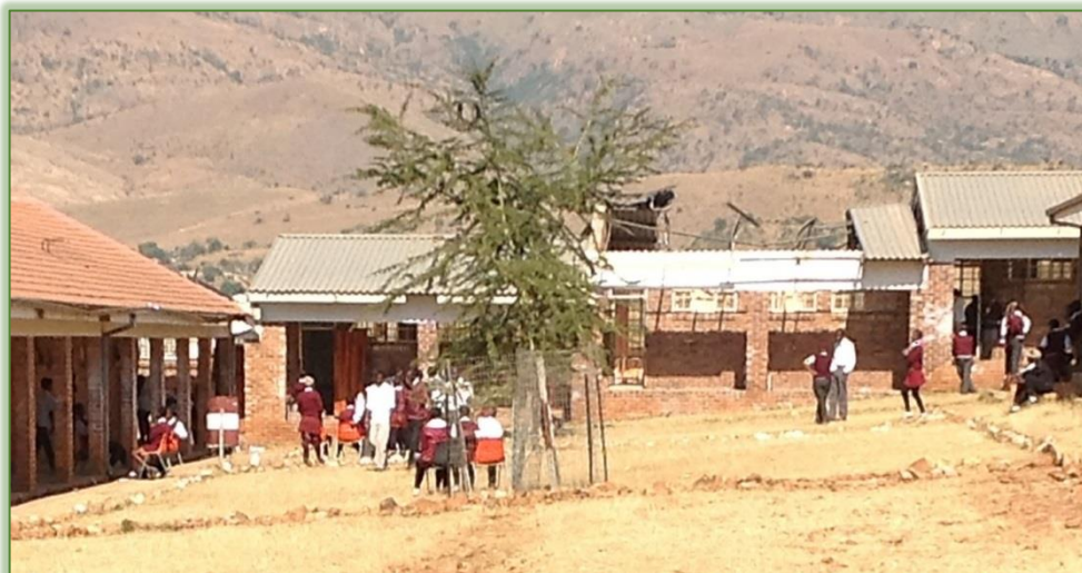
Photograph 1.1: Dilapidated school infrastructure
