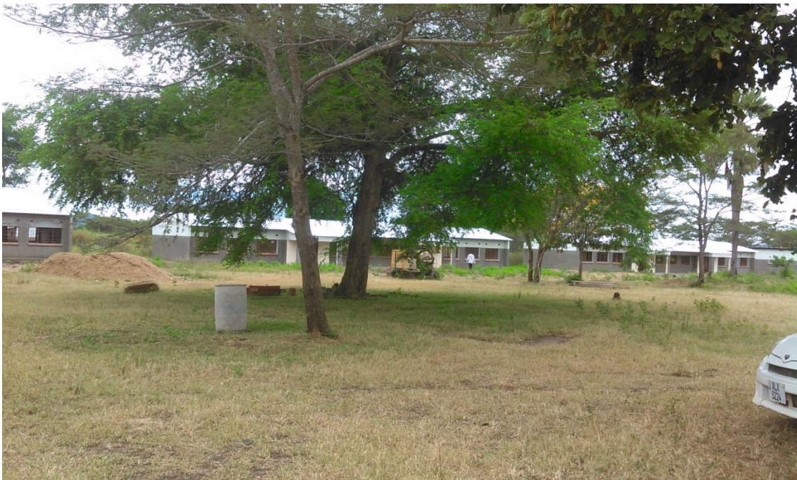
Figure 11: Classroom blocks at Munsangu School construction site
