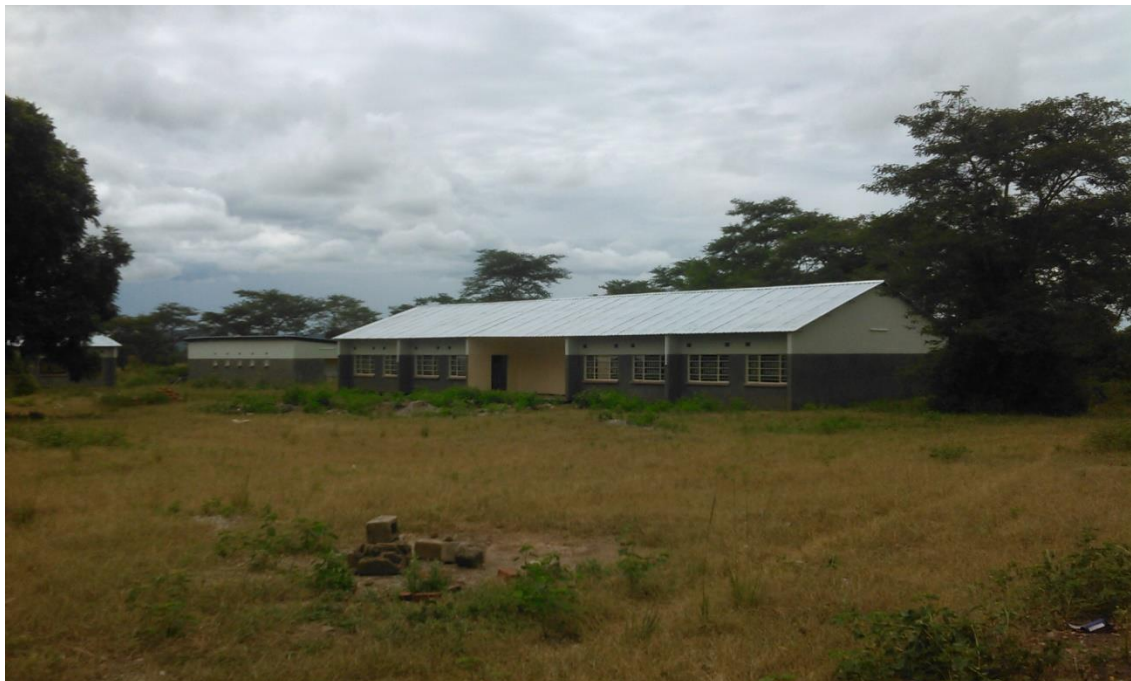
Figure 12: Wood and metal workshops block at Munsangu School building site
