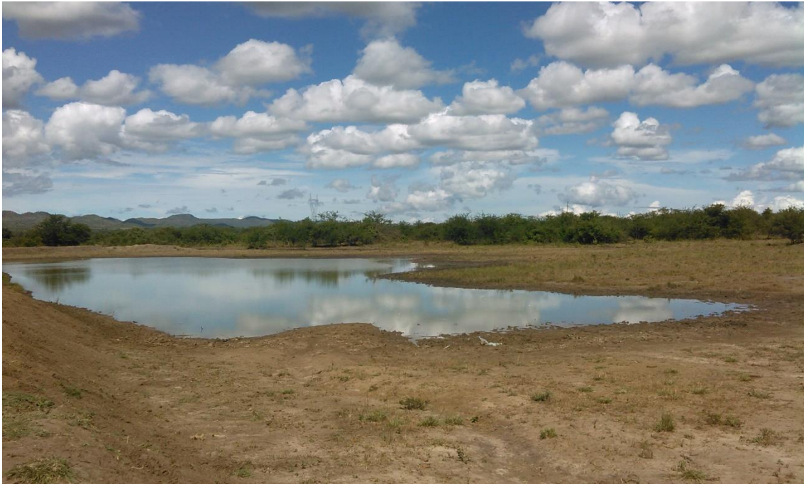
Figure 8: The Mugoto resettlement area dam
