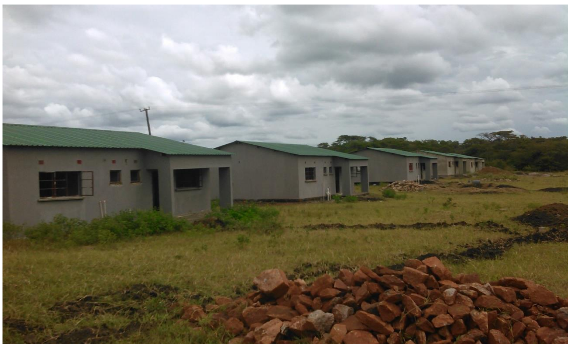
Figure 13: Teachers' houses at Munsangu School construction site
