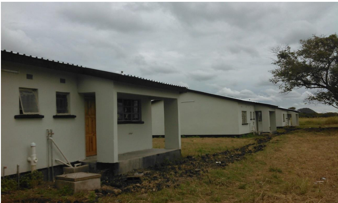
Figure 9: Houses built at Munsangu clinic construction site
