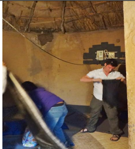
Photograph 1.4: Electricity cables used for lighting inside informal dwelling
