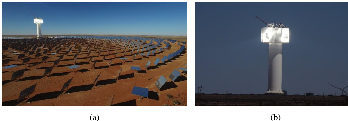
Figure 1.6: !Khi Solar One (Upington, South Africa) in operation with (a): 1 482 acre heliostat field; and (b): close-up of the 50 MW CST (Abengoa Solar, 2018)
