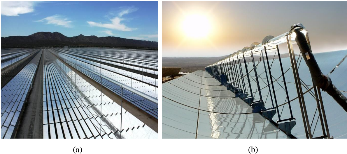
Figure 1.4(a): Linear Fresnel (TUBOSOL PE2, 2011); and (b): parabolic trough line-focus systems (Rajput, 2010)
