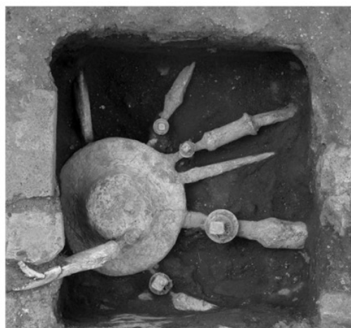
Figure 7.2: Distribution box and pipes in a) the House of the Hanging Balcony (Jansen, 2001: 28); b) the House of the Bronze Bull (Staub, 2017)
