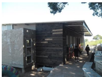
Photograph 4.26: School H’s container classrooms, school visit, 11/8/2016
