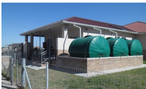
Photograph 4.37: School G's water-tanks, school visit,23/3/2016
