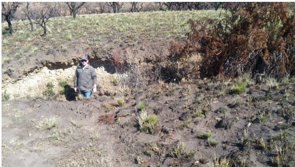
Figure 6-4: Soil piping found in the Upper Thendele camp
