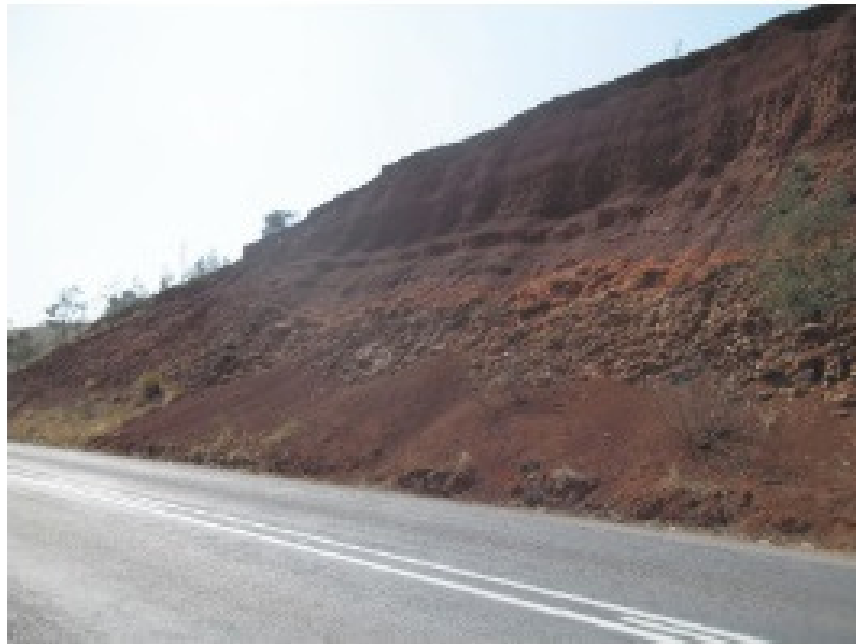
Figure 6-2: Signs of erosion on a roadside slope (Seutloali and Beckedahl, 2015b).
