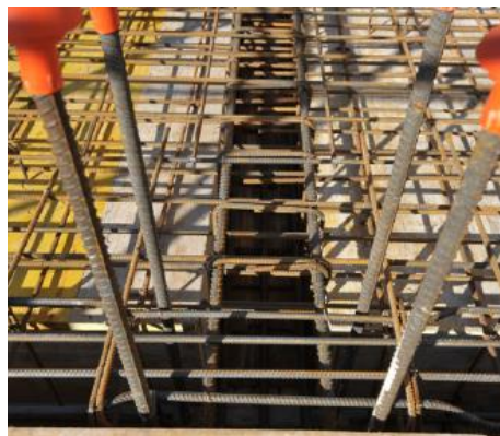
b. Central beam and slab reinforcement
