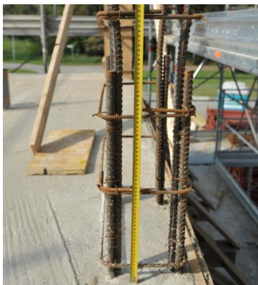
a. Column reinforcement
