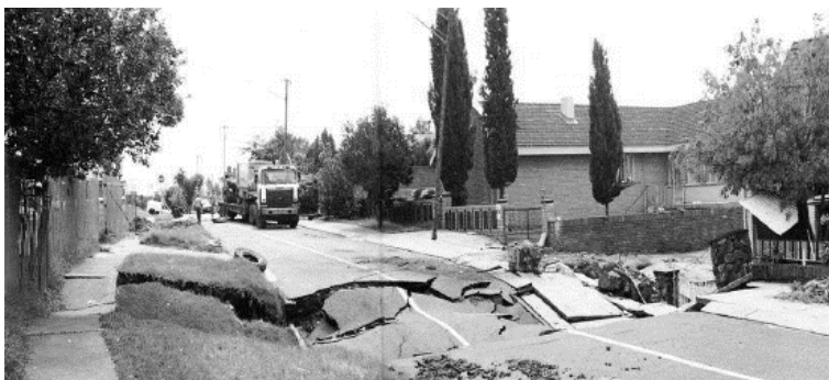
Figure 2-6: Damage to houses in Pretoria due to a sinkhole (Oosthuizen and Richardson, 2011)
