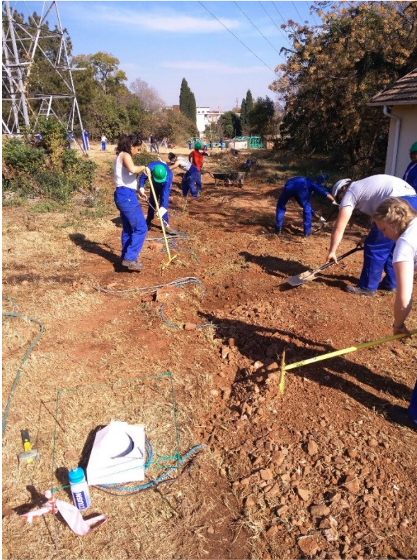
Figure 3-18: Finishing off installation
