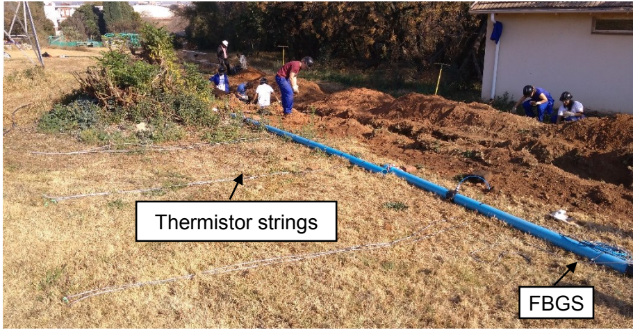
Figure 3-13: Sensor layout and levelling bottom of trench
