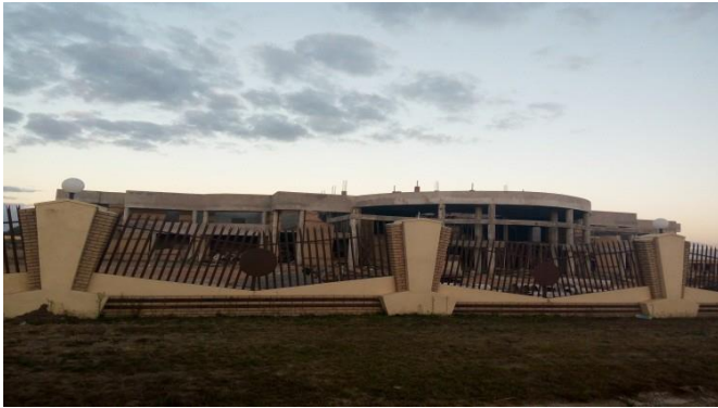
UFIC Church under construction in Chitungwiza (From own camera 16/7/17)
