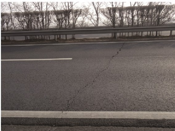
Fig. 1 – Typical transverse reflection crack.
