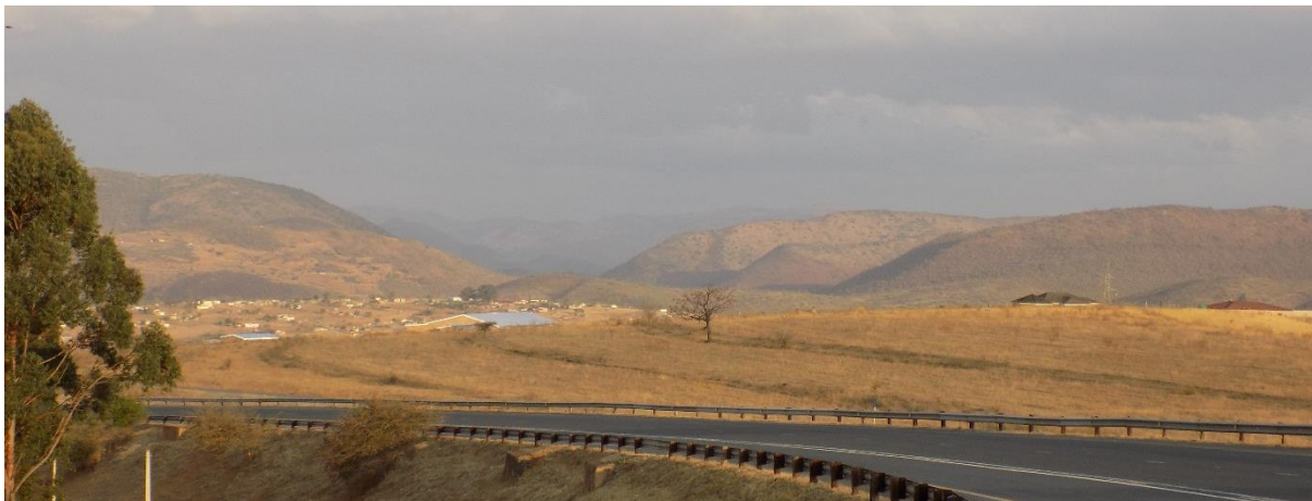
Figure 1.2 Main roadside in rural KwaZulu-Natal
