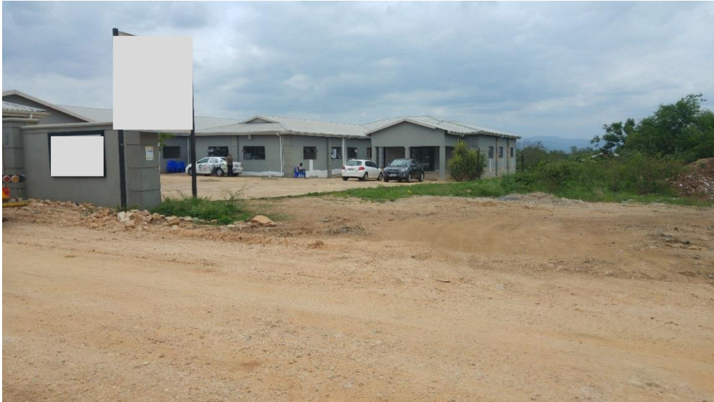
Figure 3.2 Pongola student support centre
