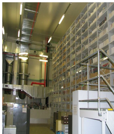
The repository building showing the multi-media area and air conditioning system
