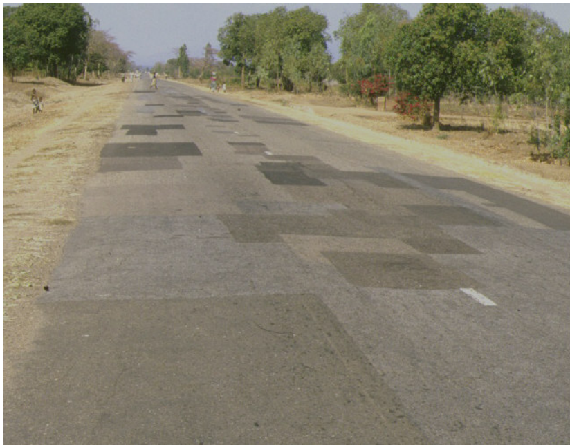
Figure 4: Changes in the condition of the surfacing causing changes in tyre wear.
