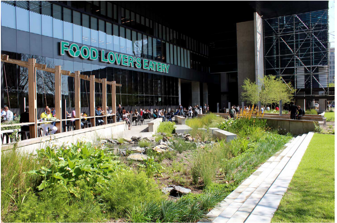
Figure5.1 Detention pond for excess roof water from The Towers roof space (Square One Landscape Architects 2017)
