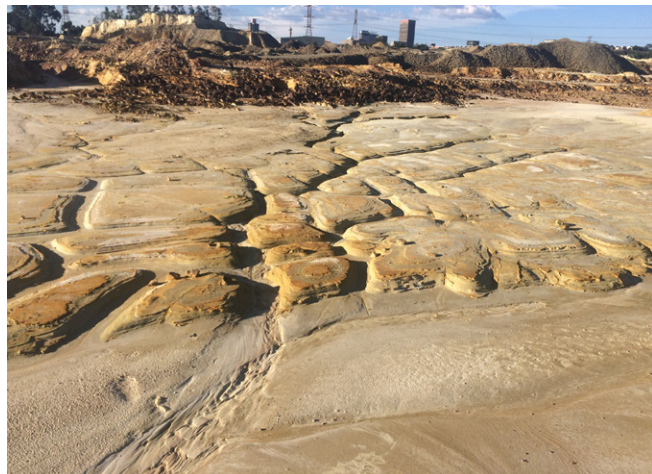
Figure3.6 Erosion caused by drainage (Author 2017)
