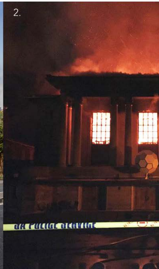
Figure 4.3 Above; Blaze taken hold in the main hall (Roos 2017)
