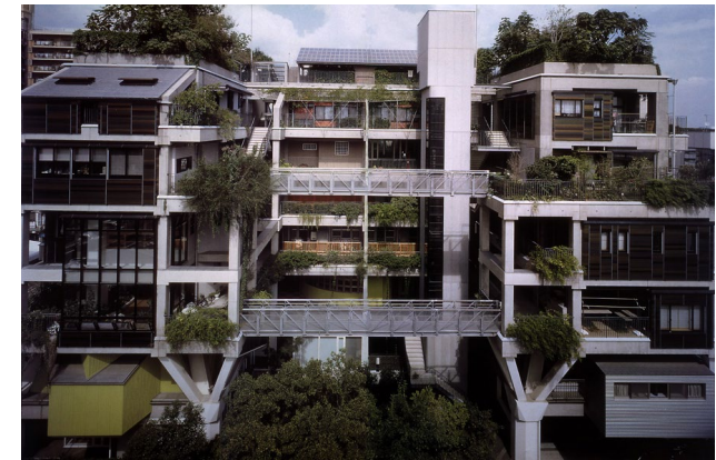
Figure 84 - View of building from adjacent buildings, indicating exposed and hidden walkways (Osaka Gas Company 1994)
