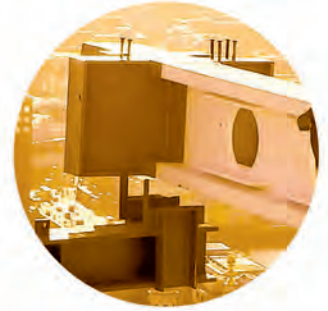
ring beam connection
