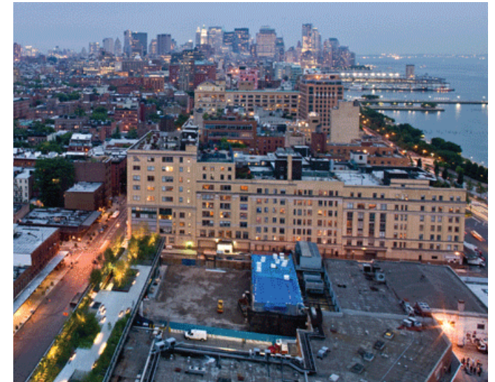
Figure 4.6: New York Highline Areal view (Open Projects, 2001)
