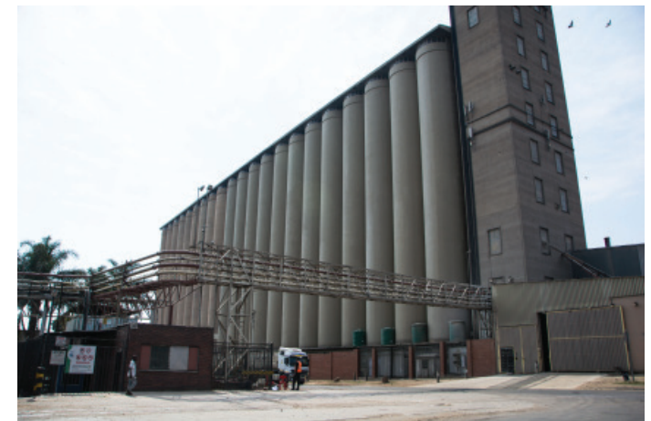
Fig. 5.8 Grain Silos with Overhead Pipes Leading to the Oil Refinement Plant (Urban Vision Group, 2017)
