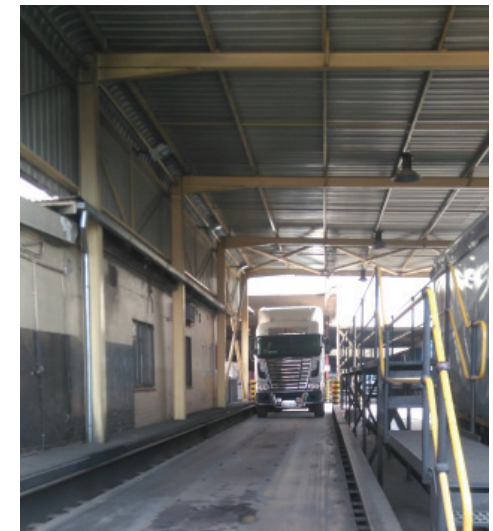
Fig. 5.11 Steel Construction as Tectonic Addition (Urban Vision Group, 2017)
