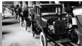
Fig. 2.7 Ford's moving Production line. Weber, A. (2013)
