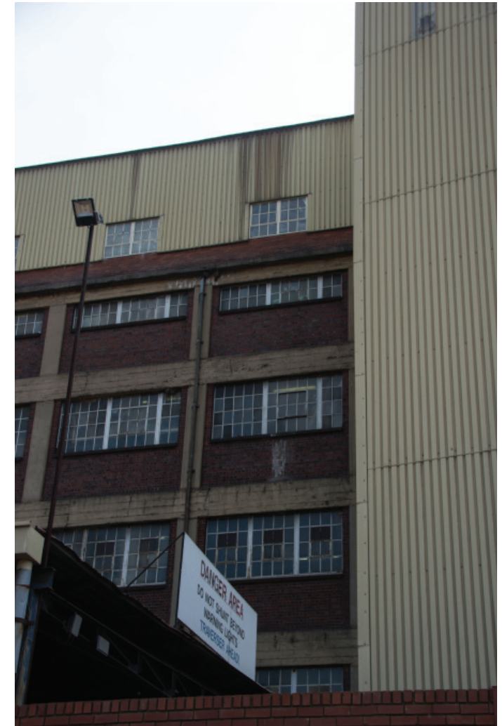
Fig. 5.2 Site photo of original facade construction (Author, 2017)
