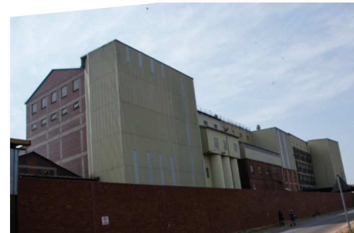
Fig. 5.6 Additive Extension to Original Structure (Author, 2017)
