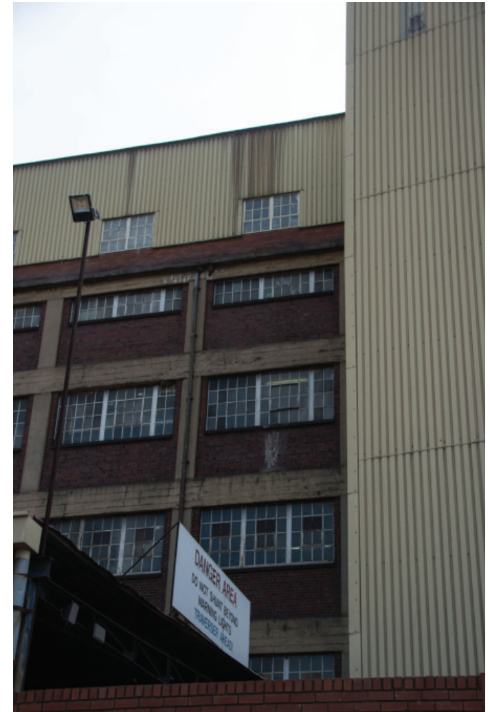
Fig. 5.2 Site photo of original facade construction (Author, 2017)
