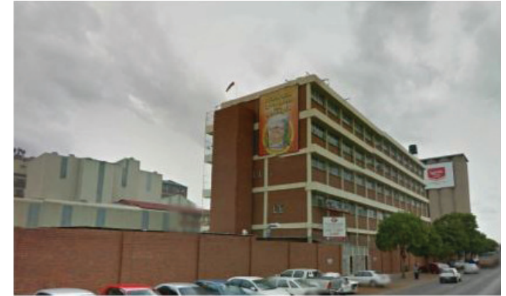
Fig. 5.7 Admin block (Google Street View, 2017)
