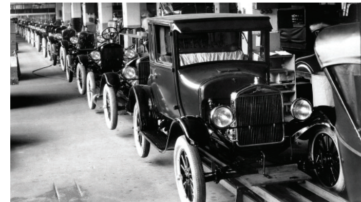
Fig. 2.7 Ford's moving Production line. Weber, A. (2013)
