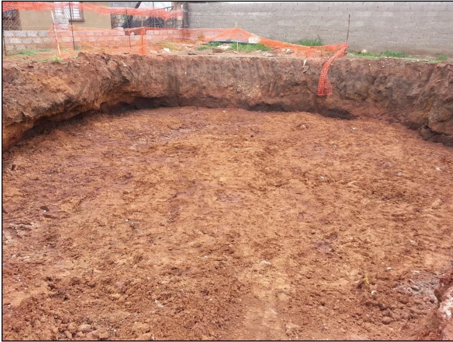
Plate C.2: Bulk excavated area backfilled to stable level.
