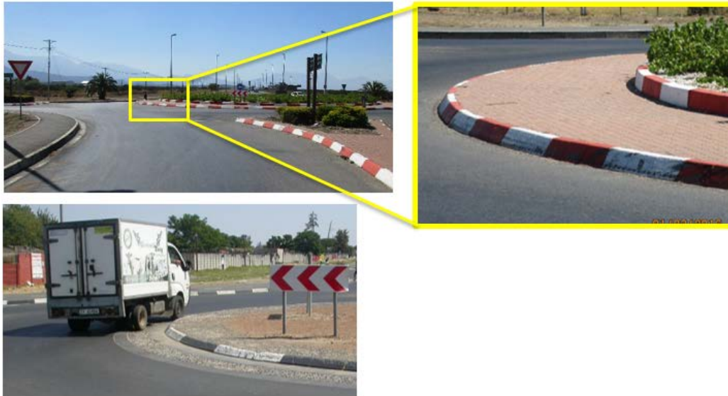
Figure 5: Truck apron not serving the purpose of design
