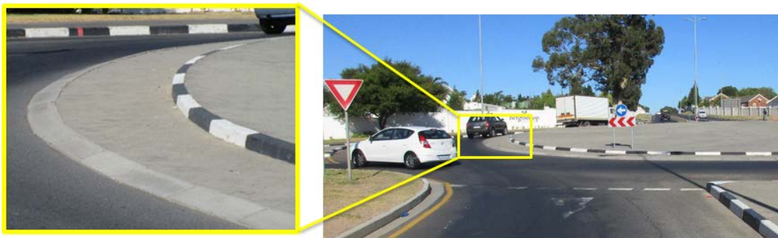
Figure 6: Truck apron with better design, but too wide circulatory lane
