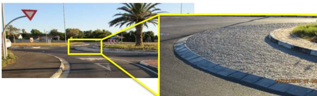
Figure 7: Truck apron with correct design for use by trucks only with a narrow circulatory roadway.
