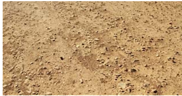
Figure 9. Oversize aggregate reflected by the 'Stoniness fixed' defect
