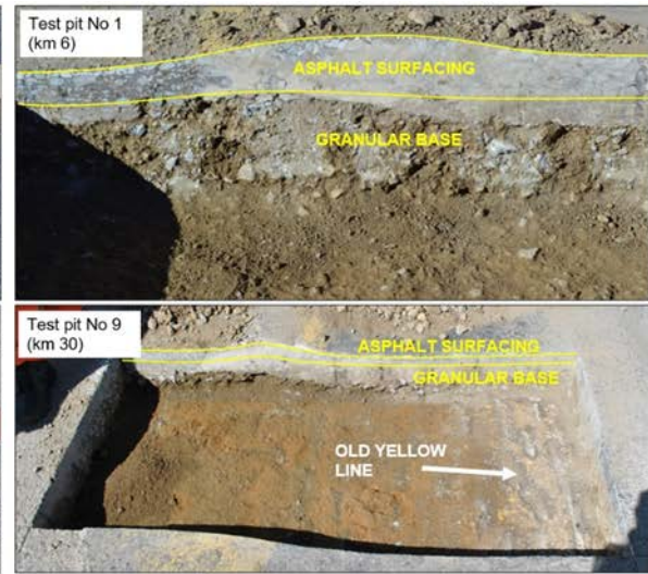
Figure 3: Profile of pavement structure where road has shoved
