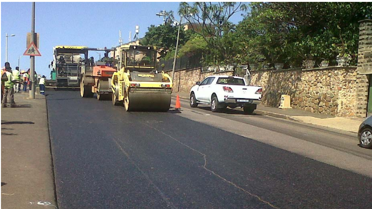
Construction of the GB5
