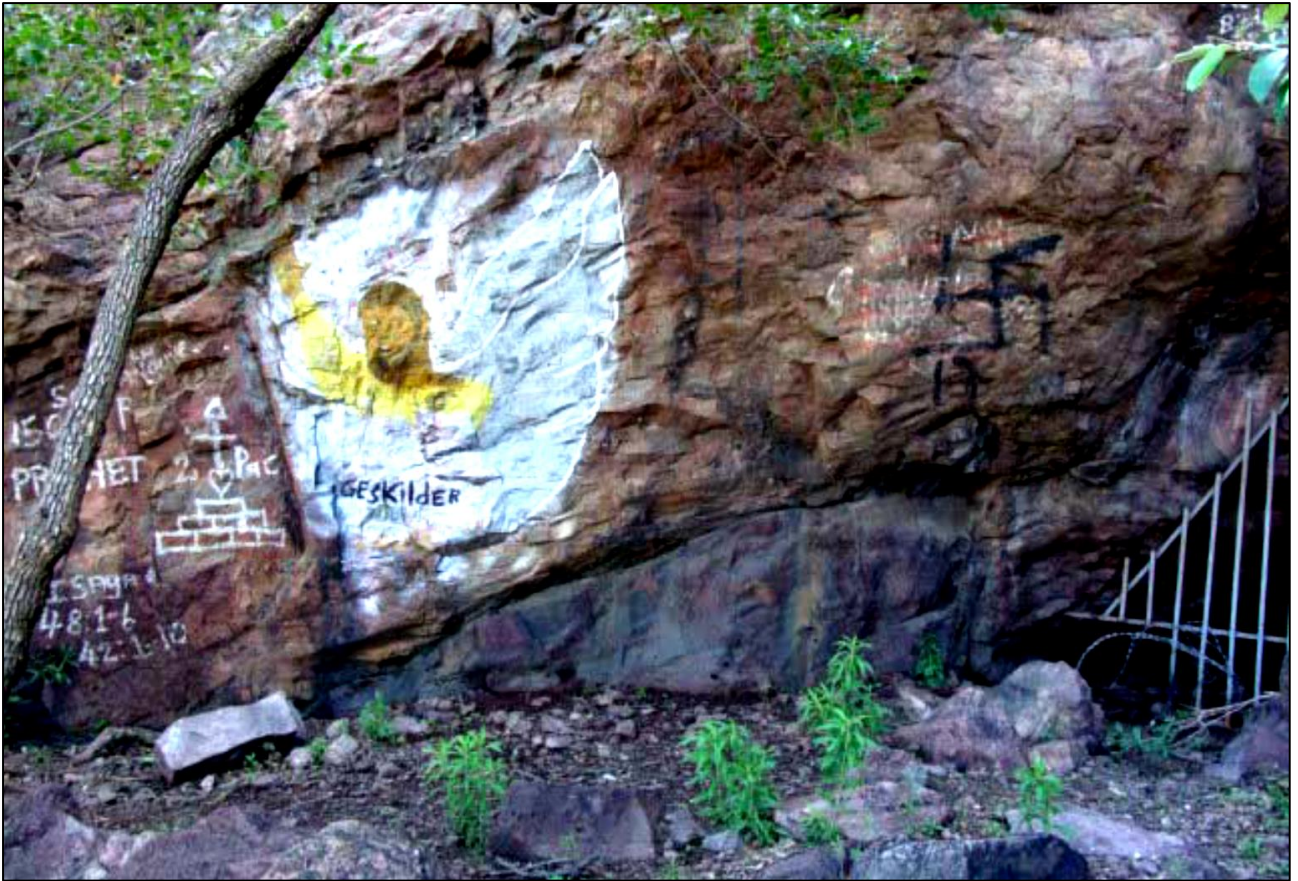
Figure 4.21: Wall at the entrance to the cave covered in graffiti
