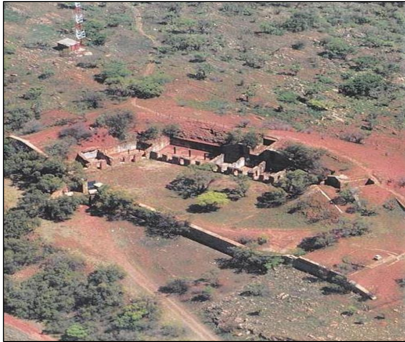
Figure 2.9: Aerial view of Fort Wonderboompoort
