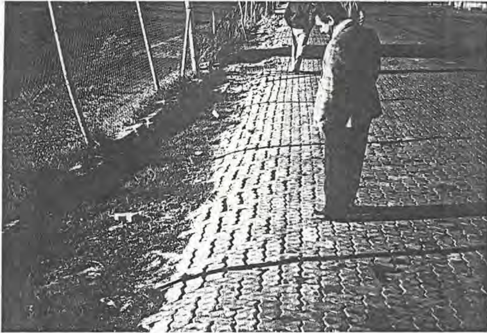
THESE BLOCKS HAVE MOVED LATERALLY BECAUSE OF A LACK OF KERBING TO CONTAIN THE BLOCKS
