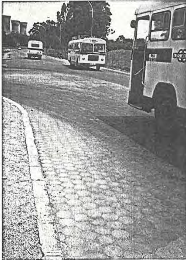
FIGURE 7.3 CIRCULAR MORTAR - JOINTED SEGMENTS IN ZIMBABWE
