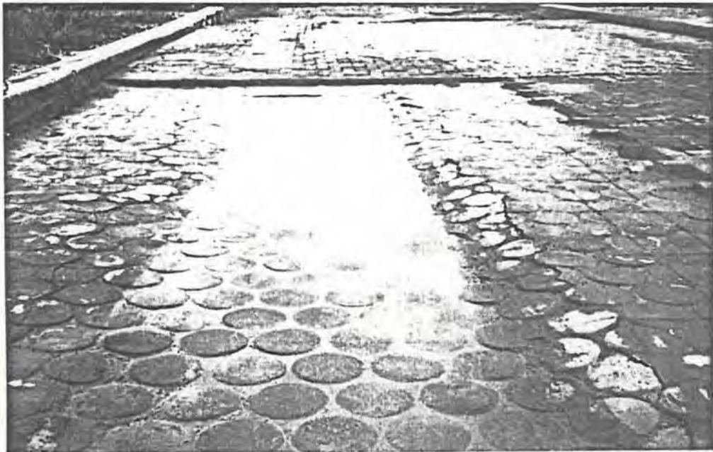
FIGURE 7.16 TEST COMPLETED SHOWING DEFORMATION AND SHEAR CRACKING ADJACENT TO TRAFFICKED AREA
