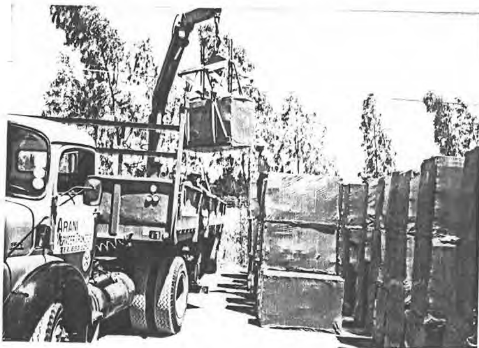
FIGURE 12.6 SHRINK-WRAPPED PALLETED BLOCKS LOADING FOR DELIVERY
