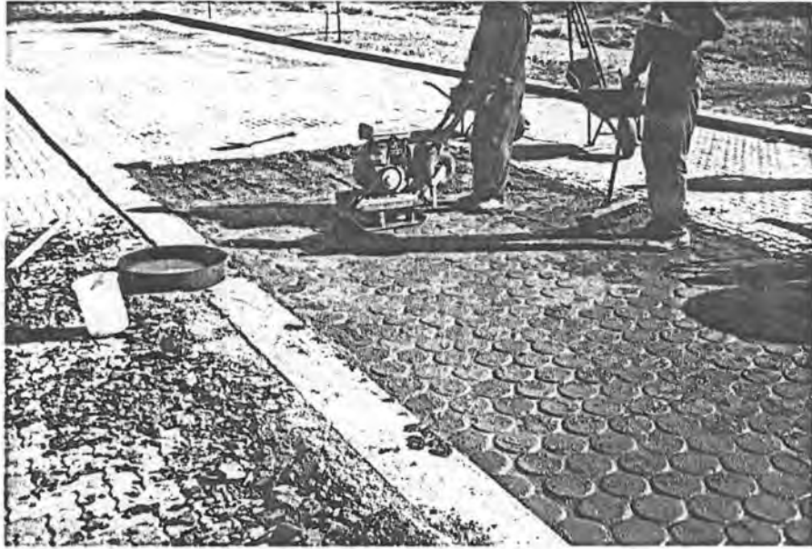
FIGURE 7.9 LIGHT VIBRATION TO INDUCE MORTAR FILLING TO COMPLETELY FILL INTERSTICES
