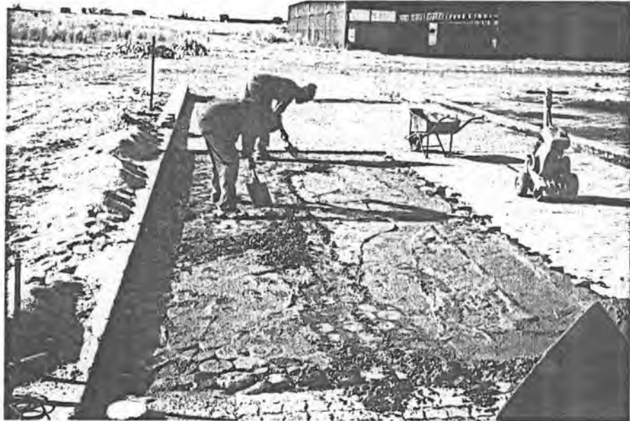
FIGURE 7.8 SPREADING MORTAR JOINTING MATERIAL
