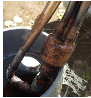
(b) Picture of underground heat exchanger in the bottom section
