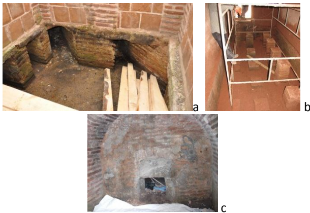
Figure 5 Hypocaust section of caldarium (a) and frigidarium (b) spaces out the bath of Suleymaniye Hospital [27] and furnace (c) of the boiler's room [29]
