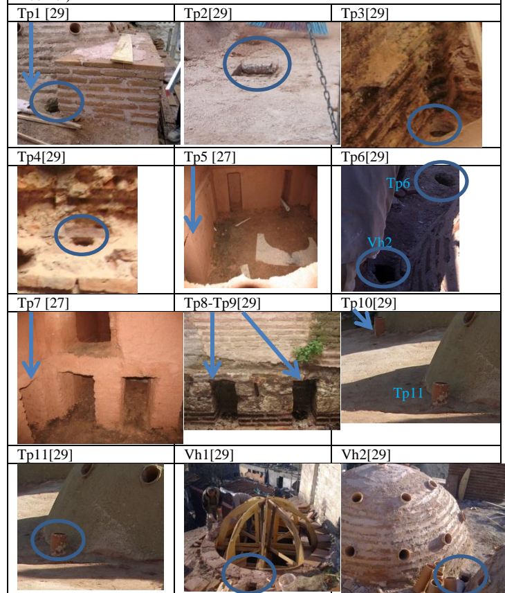
Figure 5 Hypocaust section of caldarium (a) and frigidarium (b) spaces out the bath of Suleymaniye Hospital [27] and furnace (c) of the boiler's room [29]
