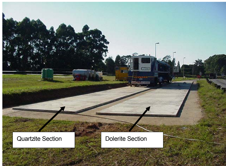
Figure 1. General view of the test site.
